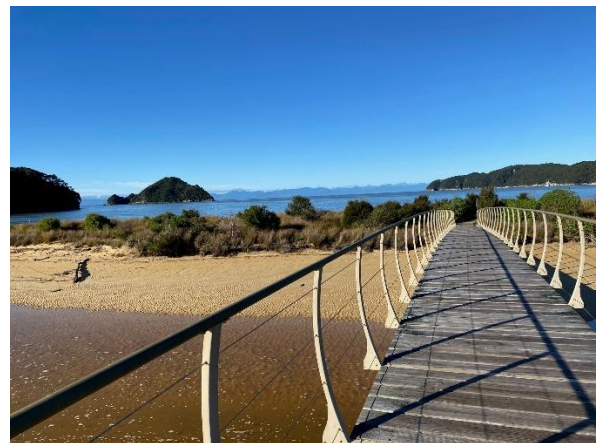
Onetahuti Bridge (Photo: J Dicks)
